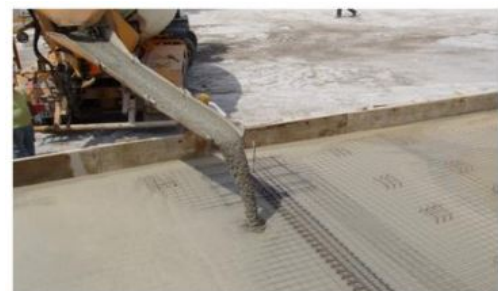
Figure 1. Casting of Self-compacting Concrete
